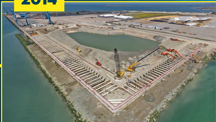
Cherbourg: creation of a 15T/sqm bearing capacity quay
