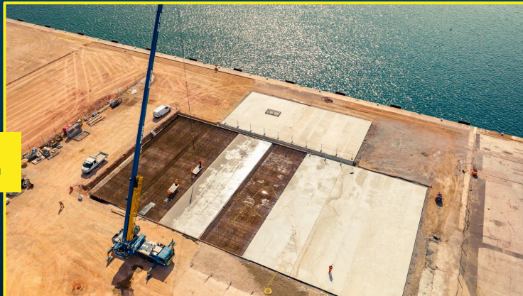
Cherbourg: partial strengthening of the heavy load quay to 27&50t/sqm min
