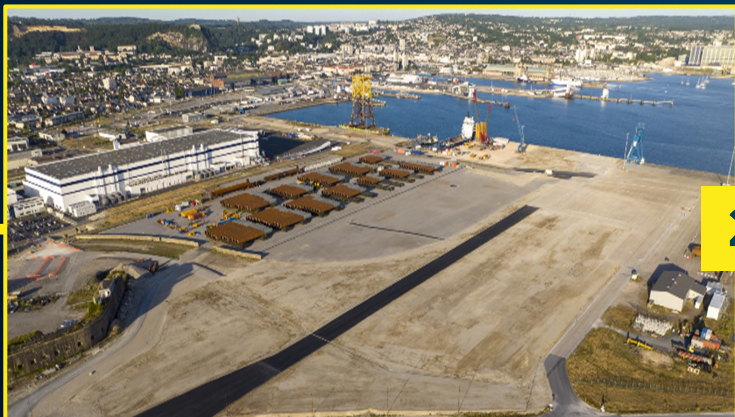
Cherbourg: fitting out an installation hub
